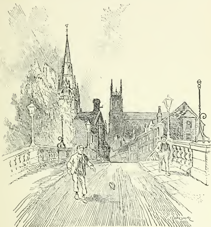
ST. MARY'S BRIDGE.
